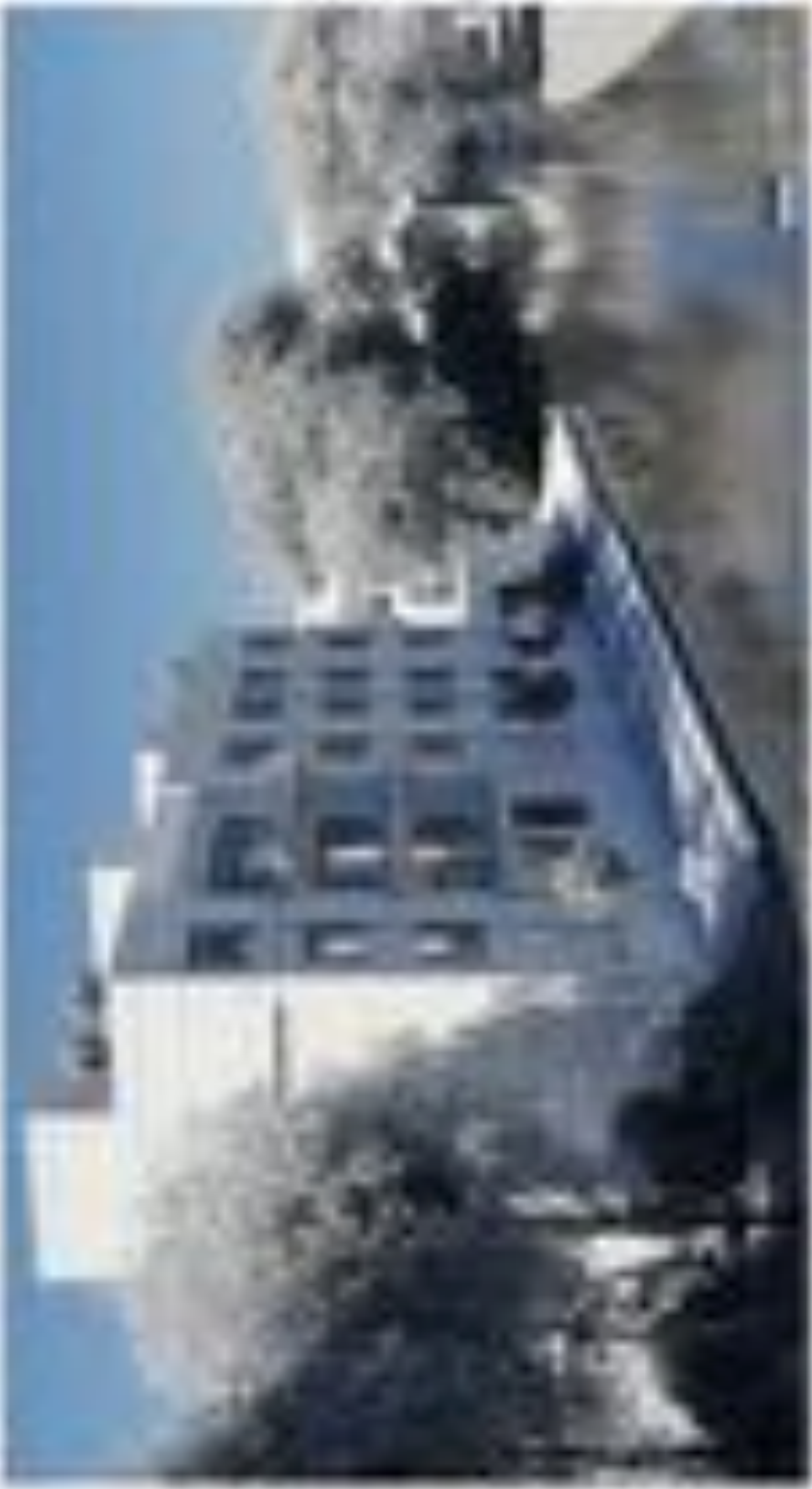
415 E FRONT - VIEW FROM THE NORTHEAST ILLUSTRATING 36" CANTILIVERED BALCONIES ON THE SECOND, THIRD AND FOURTH FLOORS
