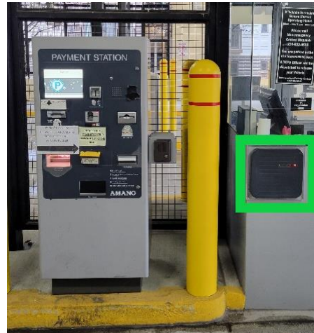
Figure 5: Shows the access card reader and intercom picture to the right. Outlined in green.
