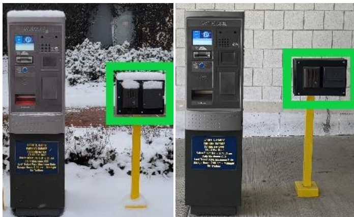
Figure 2 A, B: A(left) shows the Front St. entrance card reader and intercom, B(right) shows the State St. entrance card reader and intercom. Both outlined in green.
