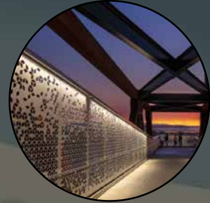
4 Bridge Accent Lighting
