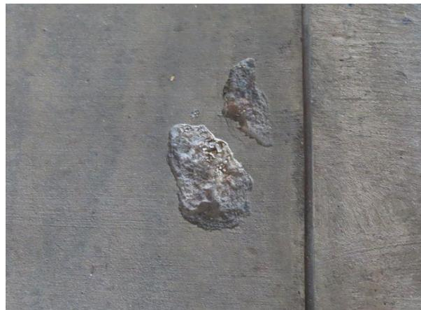
**Level 1 Slab Deterioration** — Our survey noted several areas of slab-on-grade deterioration. We recommend repairing all concrete deterioration to help prevent further deterioration and eliminate potential trip hazards.
