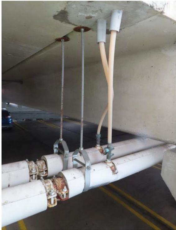
**Level 4 Center Bay Glycol Heating System** — Piping and connection of glycol heating system at underside of Level 4 in the center bay.
