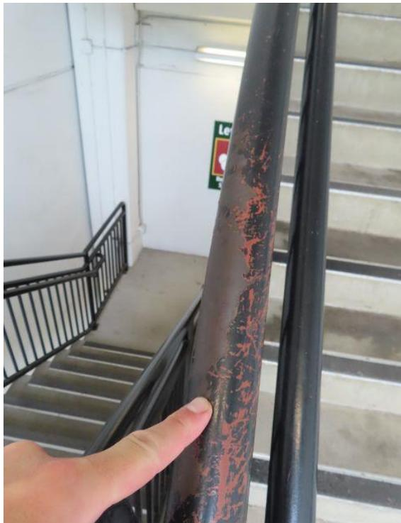
**Stair Tower Railing Deterioration** — Steel stair railings have localized areas of worn paint at areas of high traffic. We recommend cleaning and painting all steel stair railings.
