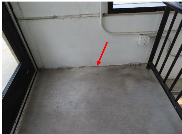
**Stair Tower Landings Missing Cove Sealant** — Stair Tower landings and elevator lobbies do not have cove sealant. We recommend installing cove sealant to limit water and salt infiltration into these joints that can lead to concrete slab deterioration.
