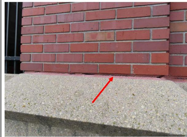
**Failed Façade Sealant** — The façade sealant around the perimeter of the structure is in poor condition with many areas of failed / crazed sealant. We recommend complete sealant replacement.
