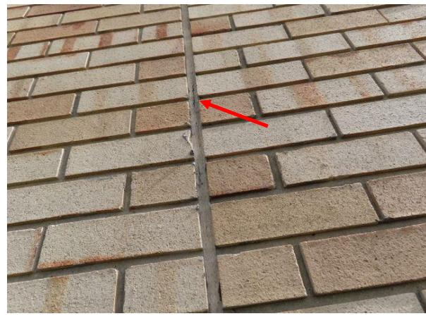
**Failed Façade Sealant** — Numerous failures in the façade sealant. The exterior façade sealant is near the end of its useful life. We recommend façade sealant be replaced in years 4 or 5 of the repair plan.
