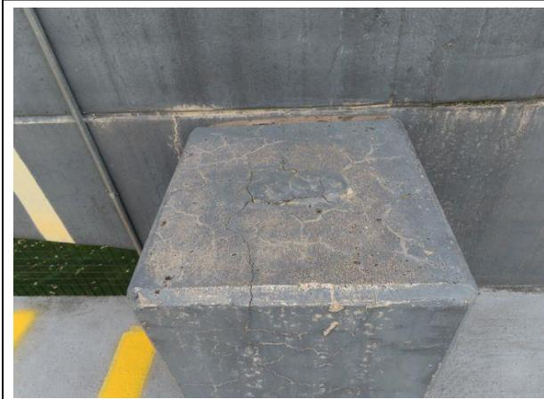
**Level 4 Concrete Column Cracking** — Concrete column on Level 4 with map cracking that may be Alkali-Silica-Reaction. We recommend installing a protective coating to limit water infiltration into these columns and slow concrete deterioration.
