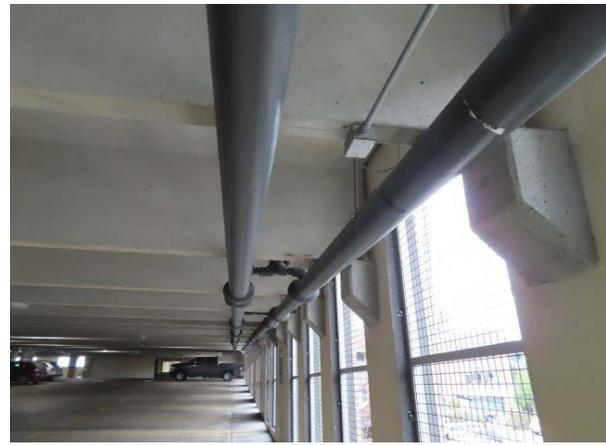
**Piping for Level 4 Heating System** — Underside of Level 4 east bay showing the piping for the glycol heating system.
