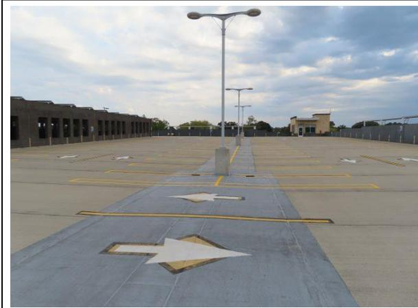
**Traffic Bearing Membrane Between Center / West Bays** — Cast-in-place concrete washes between west bay and center bay are covered with a traffic bearing membrane on all supported levels.
