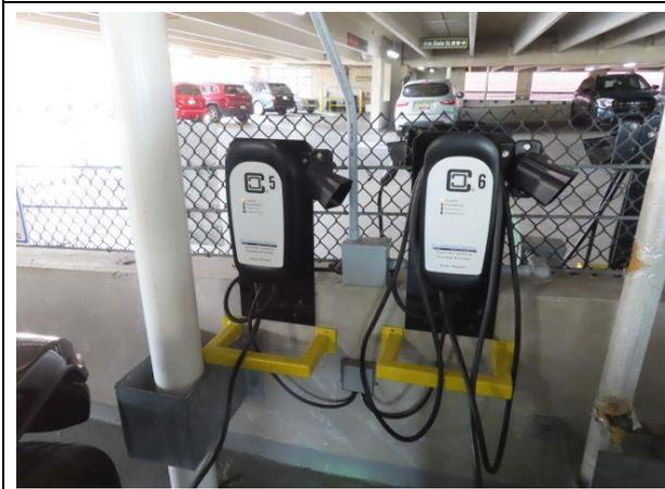
**Typical Electric Vehicle Charging Station** — EV charging stations are typically found at the south end on the east bay on the supported levels.
