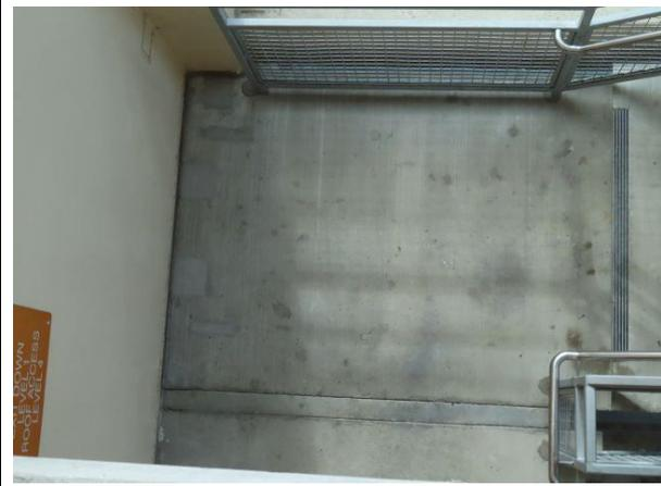
**Stair Tower Landing** — Close-up photo of stair landing showing unsealed tooled joints. All landings and elevator lobbies have unsealed joints. We recommend sealing these joints and installing a traffic bearing membrane to limit water and salt infiltration that can lead to future concrete deterioration.
