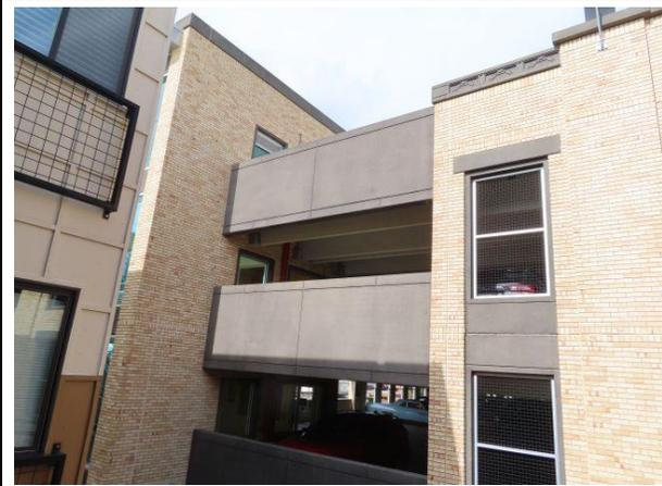
**South Façade at Stair Tower** — South façade at southwest stair / elevator tower. Photo shows precast spandrel beams with no in-laid brick.
