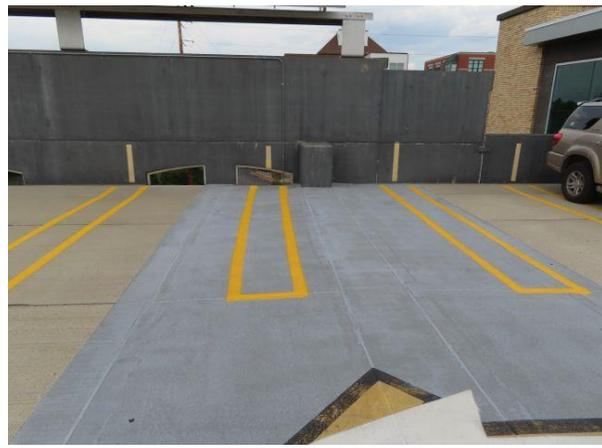
**Crossover Traffic Bearing Membrane** — Traffic bearing membrane installed over one of the crossovers on Level 4. All supported levels of the structure have traffic bearing membranes installed over the cast-in-place washes at these crossovers.
