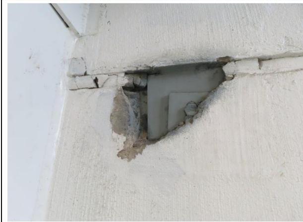
**Missing Grout Pocket** — Approximately ½ of the grout is missing at this location at a precast wall panel at the southeast stair tower. We recommend patching all missing / damaged grout pockets to protect the steel connections behind them from future deterioration.
