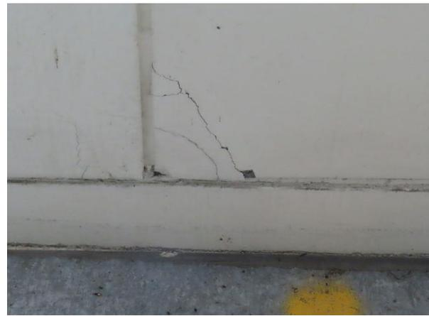
**Perimeter Wall Cracking** — Wall cracking at perimeter spandrel panels. We recommend repairing all cracked / deteriorated wall panels.
