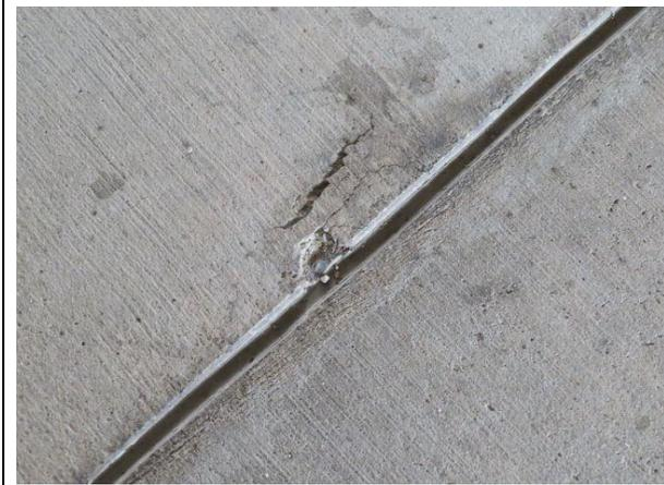
**Supported Level Slab Deterioration** — Our survey noted many areas of supported level concrete slab deterioration that we recommend be repaired. Most of the slab deterioration at the supported levels is located along the joints. After concrete slab repairs are completed, we recommend traffic bearing membrane strips (similar to Level 4) be installed at all lower-level tee-to-tee joint sealants.
