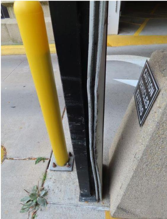
**North Entry / Exit Roll Down Gate** — The metal tracks at the north entrance roll down gate have been damaged. The City may want to consider replacing this metal track for the roll down gate. No costs have been included for this work.
