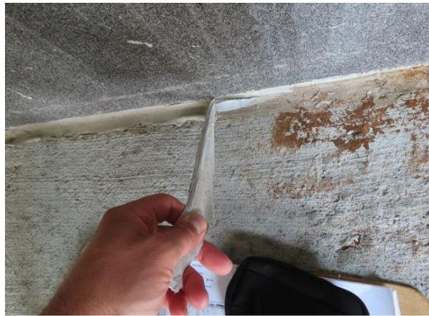
**Failing Sealant** — Previous repairs installed a skim coat of sealant over the previous sealant at the stair towers instead of removing and replacing the sealant. We recommend all stair tower sealants be replaced.
