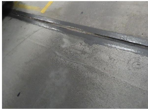
**Worn Traffic Coating on Level 1 to Level 2 Ramp** — We recommend repairing and recoating all existing traffic bearing membranes to keep them functioning as intended and protect the underlying concrete elements from future deterioration.
