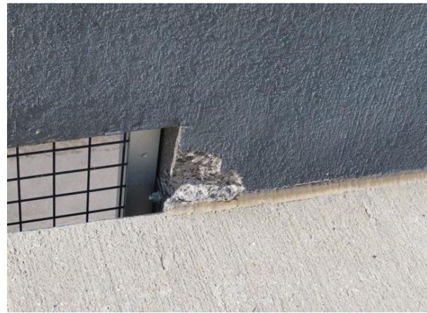
**Perimeter Wall Damage** — Concrete wall damage on Level 4 perimeter walls that may be the result of snowplow damage.
