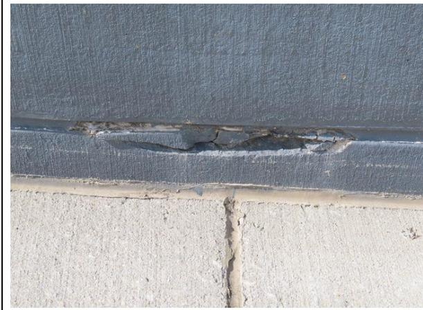
**Perimeter Wall Deterioration** — Concrete wall deterioration on Level 4 perimeter. This wall deterioration / damage appears to be the result of snowplow damage.
