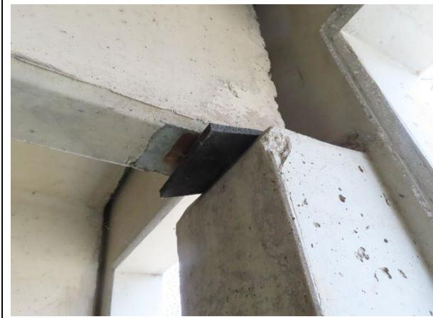
**Shifted Bearing Pad** — Our survey noted several shifted bearing pads under precast double tee elements. We recommend monitoring these shifted bearing pads to make sure they do not worsen.
