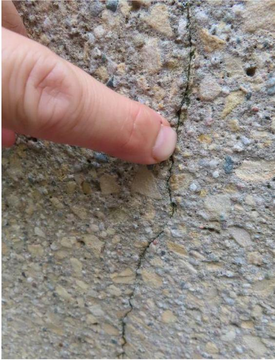
**Precast Spandrel Panel Cracking** — Close-up photo of the spandrel panel cracking.
