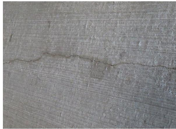
**Level 1 Grade Slab Cracking** — Level 1 slab-on-grade cracking. We recommend monitoring this cracking and as long as it does not become displaced / settle no work is required.
