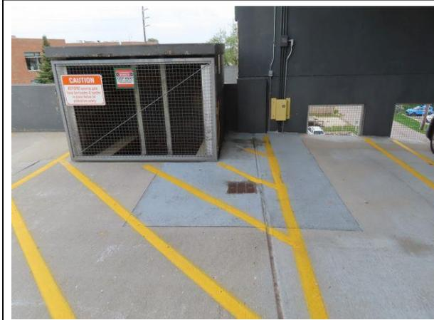
**Snow Dump and Floor Drain** — Snow dump from the Roof Level and a floor drain with a traffic bearing membrane around it. The snow dump drops snow down two levels and drops the snow onto the east alley.
