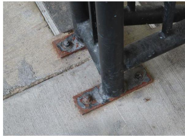
**Stair Tower Railing Deterioration** — Steel stair railings have localized areas of deterioration typically at the railing anchor posts. We recommend cleaning and painting all steel stair railings.
