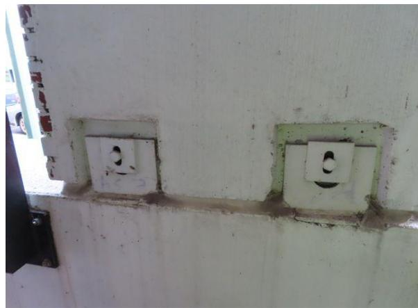
**Precast Spandrel Panel Steel Connection Plates** — The exposed steel plates have been painted and appear to be in good condition.
