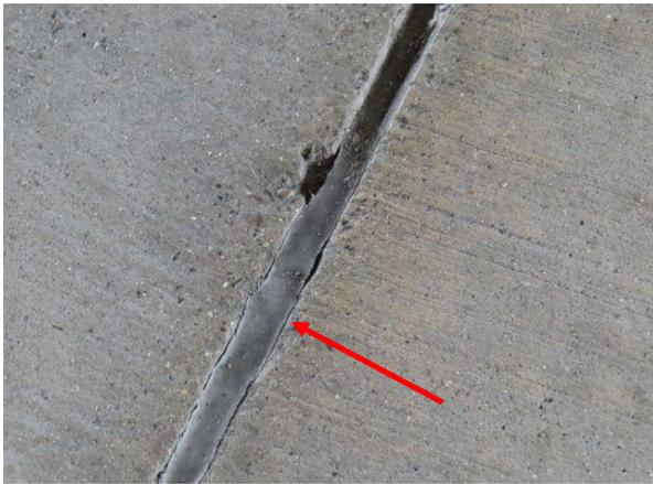
**Failed Joint Sealant** — The joint sealant has failed at this location.
