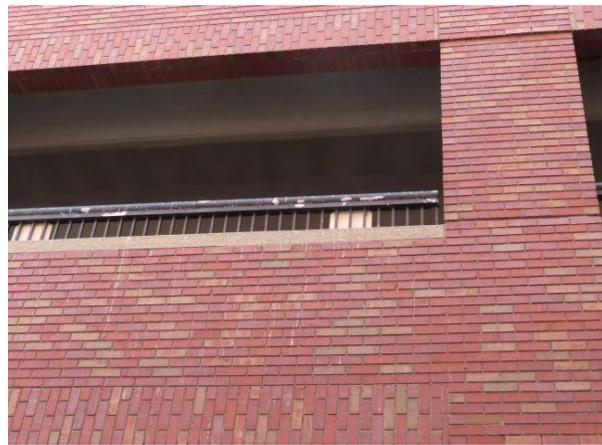
**Perimeter Railings Peeling Paint** — The railings / fences around the perimeter of all levels are painted metal. Several areas of peeling / missing paint were observed. We recommend cleaning / painting these railings.
