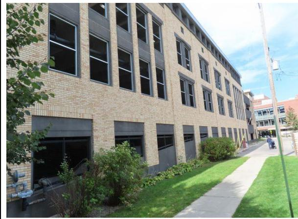
**East Façade** — Façade on the east elevation of the structure consists of precast concrete panels with in-laid brick and aluminum frames with powder coated mesh panels at the window openings.
