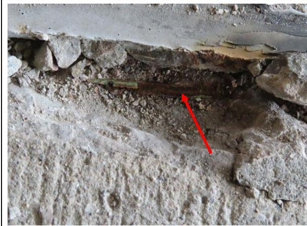
**Supported Level Slab Deterioration** — Another location of slab deterioration along a tee-to-tee joint. The deterioration at this location is likely due to moisture / chloride intrusion from failed joint sealant. The concrete has spalled exposing the steel reinforcement which has corroded.
