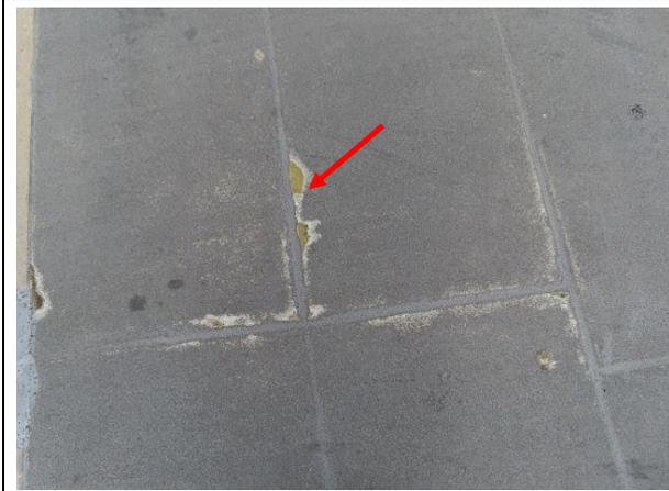
**Level 4 Traffic Coating Damage** — Worn traffic coating was observed at the crossover at this location. See above for repair recommendation.
