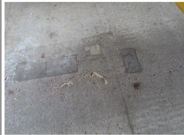
**Level 1 Slab Deterioration** — Our survey noted several areas of slab-on-grade deterioration that we recommend be repaired.
