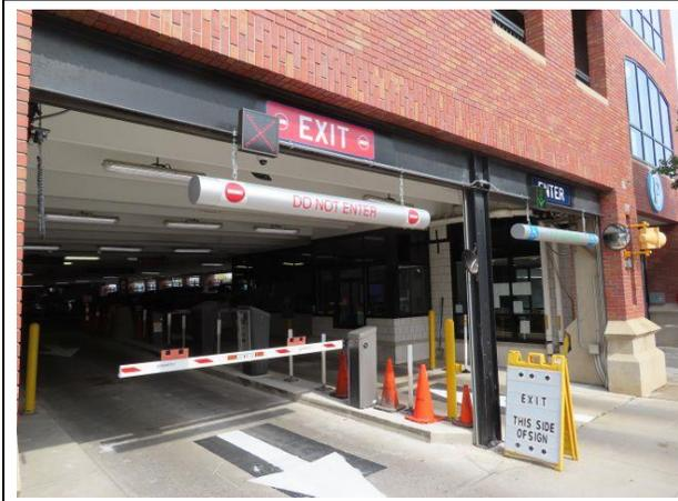
**South Entry / Exit PARC Equipment** — This photo shows the parking access and revenue control (PARC) equipment at the south entry / exit.
