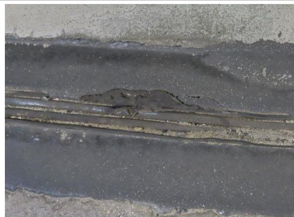
**Expansion Joint Deterioration** — The expansion joint at the center ramp between the supported level and grade level is cracked and in need of repairs / replacement maintenance.
