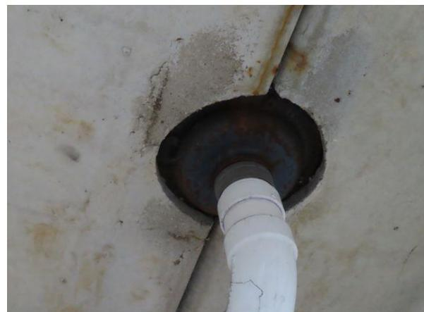
**Floor Drain Concrete Slab Deterioration** — Concrete slabs are deteriorating around rusting floor drains. We recommend localized floor drain replacement and concrete slab repairs.
