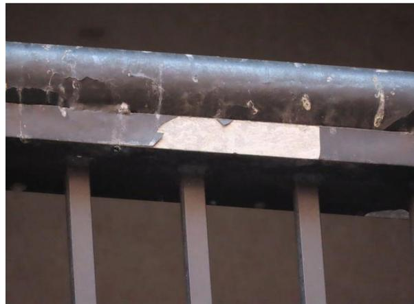
**Perimeter Railings Peeling Paint** — Close-up photo of the peeling paint.
