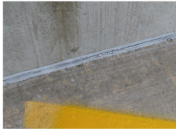
**Cove Joint Sealant** — Failed / damaged cove joint sealant was observed throughout the structure. It appears that the cove sealants have exceeded their anticipated useful life. We recommend replacing all cove joint sealants to protect the underlying structural elements from future deterioration.
