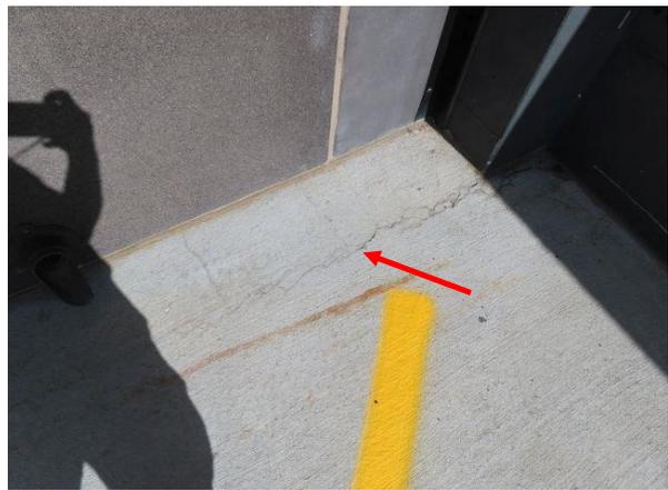
**Slab Cracking** — Open slab cracks were noted throughout the supported levels. We recommend open slab cracks be routed and sealed.
