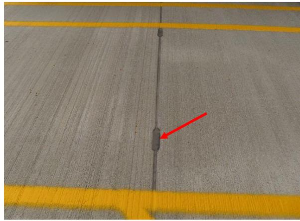
**Typical Tee-to-Tee Joint Sealant** — Sealant at typical joint between two (2) precast double tee sections. Since the structure is pre-topped the sealant joints are larger at each shear connector (red arrow). The joint sealants are generally in good condition but are near the end of their useful life and will likely need to be replaced in the next 4 to 5 years.
