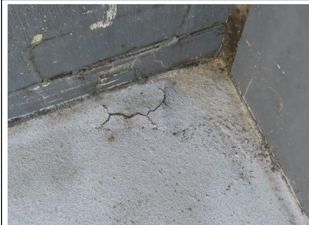
**Traffic Bearing Membrane Deterioration** — Traffic bearing membrane damage that needs to be repaired.
