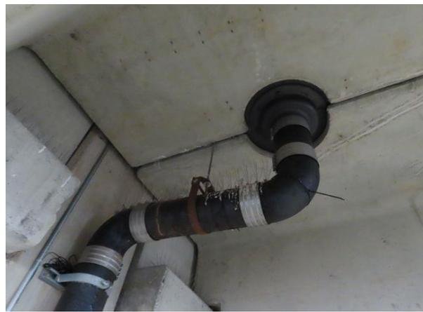
**Floor Drain & Piping** — Typical supported level floor drain with cast-iron piping. This piping may require future replacement maintenance as it corrodes.
