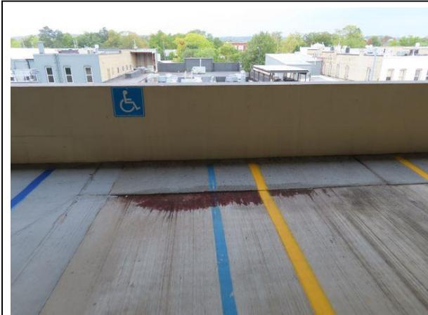
**Ponding Water Location** — Location of previous ponding water. We recommend installing supplemental drains at locations of standing water.
