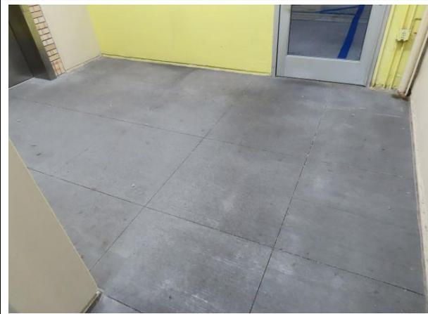
**Elevator Lobby** — Typical elevator lobby at southwest stair tower. The concrete slab has sawcut joints that are unsealed that we recommend be routed and sealed. We also recommend a traffic bearing membrane be installed to help protect against future deterioration.
