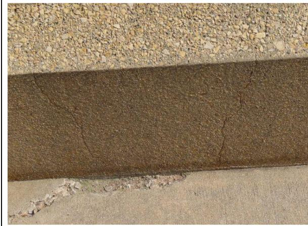
**Precast Spandrel Panel Cracking** — Our survey noted many areas of the concrete spandrel panels along the perimeter with cracking. We recommend monitoring this cracking to determine if it worsens. The city may want to consider routing and sealing these cracks to limit water and salt infiltration.
