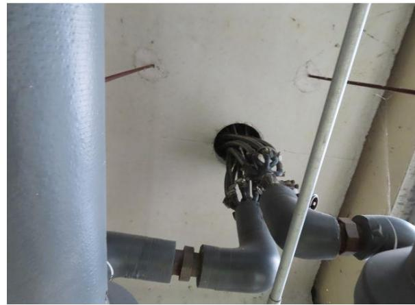
**Glycol Heating System at Level 4 East Bay** — Underside of Level 4 east bay showing the glycol heating system for the east bay. This system is only on the Level 4 east bay and is used to melt snow and ice on the sloped bay.
