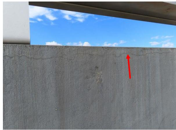
**Perimeter Wall Cracking** — Perimeter spandrel wall cracking. We recommend monitoring this cracking to determine if it worsens.
