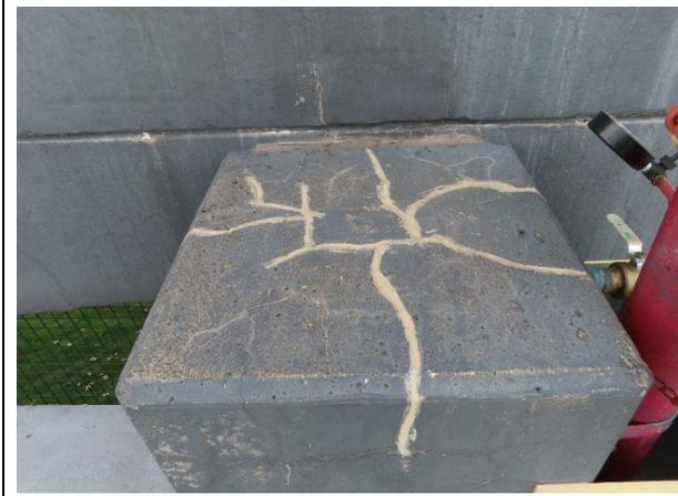
**Level 4 Concrete Column Cracking** — Another Level 4 column showing similar cracking like the column above where some of the cracking has been sealed. However, additional cracking is now evident. A membrane is the best way to cover the cracking and limit water infiltration.
