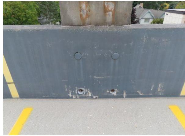
**Missing Wall Coverings** — Missing spandrel panel lifting hole covers. We recommend replacing these covers to limit water from entering the panels through these holes.
