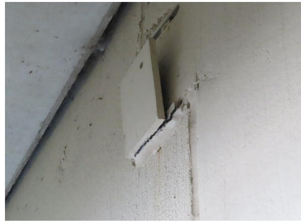
**Wall Connection Plate Repair** — Perimeter wall connection plate that is no longer connected. We recommend re-connecting plate.
