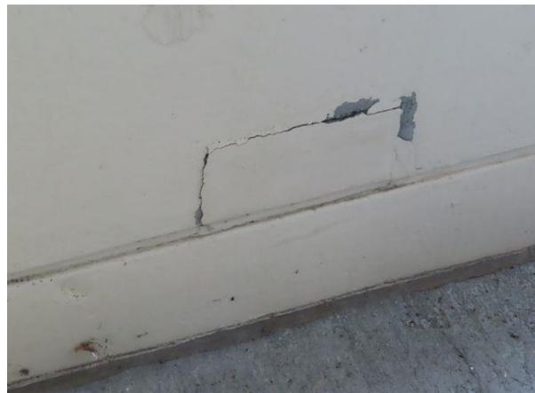
**Cracked Grout Pocket** — Perimeter spandrel panel grout pocket that is cracked and loose. We recommend replacing all cracked / loose grout pockets.
