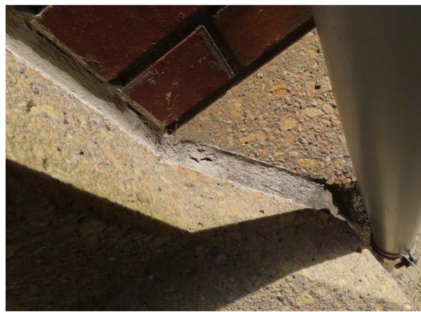
**Failed Façade Sealant** — The façade sealant around the perimeter of the structure is in poor condition with many areas of failed / crazed sealant. It appears that these sealants have exceeded their useful life. We recommend complete sealant replacement.
