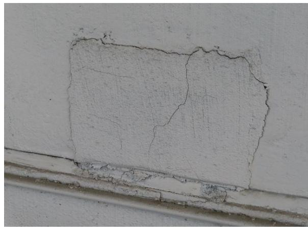
**Cracked Grout Pocket** — The grout has cracked at this location. We recommend patching all cracked / damaged grout pockets to protect the steel connections behind them from future deterioration.
