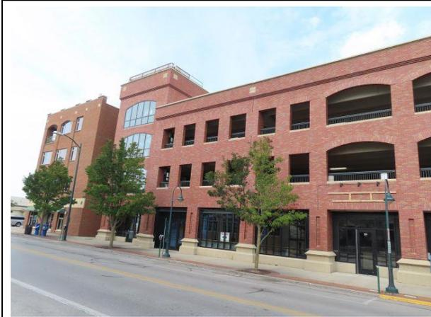
**South Facade** — The structure consists of three (3) supported levels and one (1) grade level of parking. Patrons move between levels via the center ramp. The outer parking bays are flat. The façade consists of precast concrete panels with thin brick. Painted metal railings are provided at the openings. Aluminum framed glass storefront systems are provided at the stair towers and at the occupied retail/office space at Level 1 at the south elevation.
