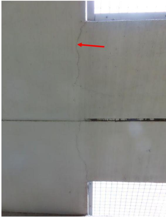
**Perimeter Wall Cracking** — Lower-level perimeter spandrel panel cracking. We recommend monitoring this cracking to determine if it worsens.
