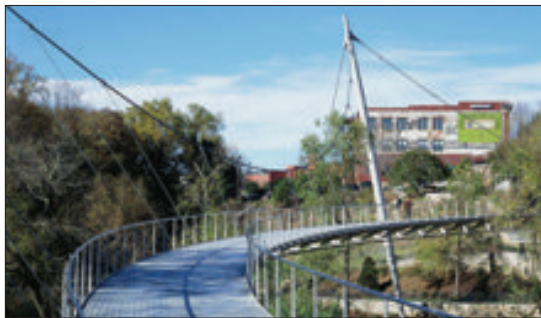
Greenville, South Carolina's curving pedestrian bridge, known as the Liberty Bridge at Falls Park on the Reedy, is listed as a landmark attraction by cityprofile.com. Designed by schlaich bergemann und partner, the bridge showcases the potential of a unique bridge to draw attention to this area of Traverse City.
