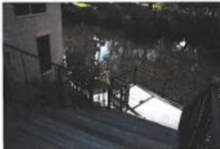
River Access Staircase at Uptown Court - Existing
