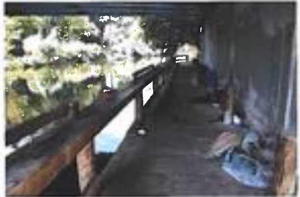
Boardwalk at Union Street Bridge - Existing
