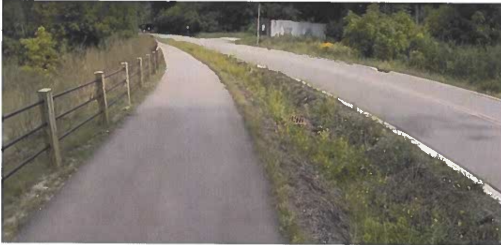
Figure 40. Lake Street Pervious Concrete Intersection and Bioswale. Image from https://www.youtube.com/watch?v=Qxf3T2oGqGM
