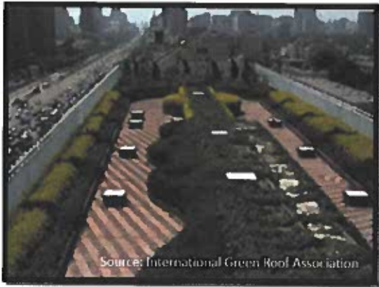
Figure 24. Intensive Green Roof System
