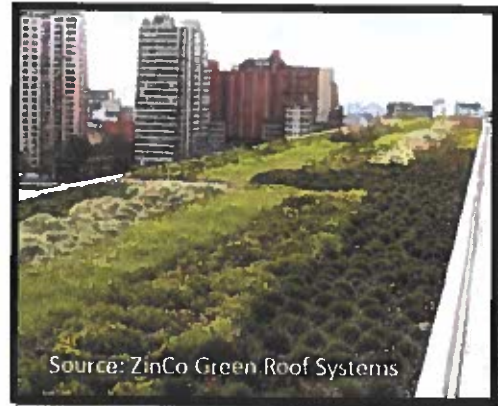
Figure 23. Extensive Green Roof System
