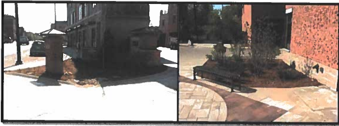
Figure 46. Rain Gardens Constructed In 2017 by Uptown Development TC, LLC
