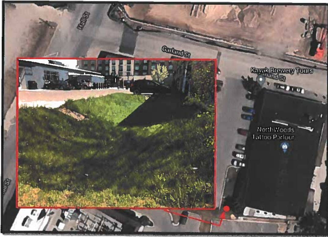
Figure 51. Existing Infiltration Basin by NorthWoods Tattoo Parlour
