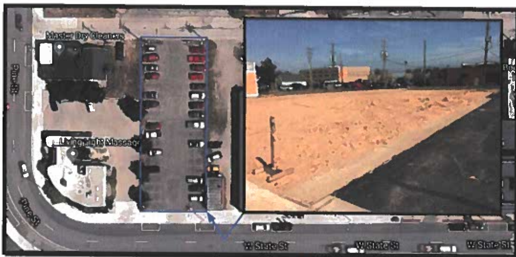
Figure 69 - Construction Site without Silt Fence
