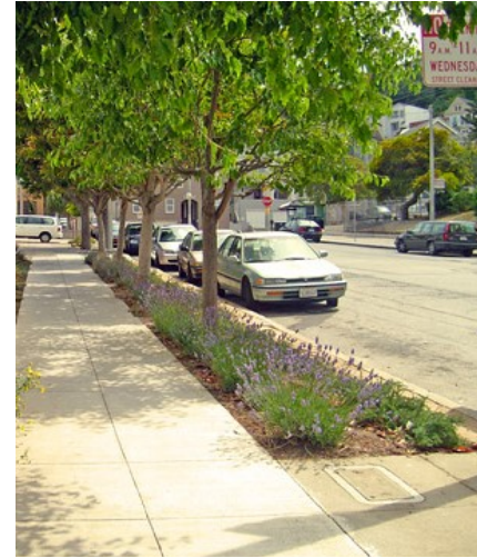
Figure 10. Contiguous open tree & landscape bed Photo: sfbetterstreets.org
