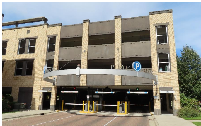
Old Town Parking Structure
