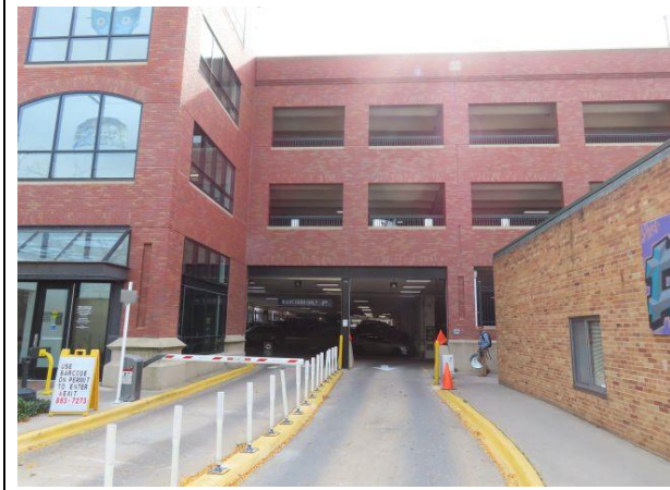
North Facade — North façade and entry / exit to the structure. This along with the south entry / exit are the two ways patrons can enter / exit the structure.
