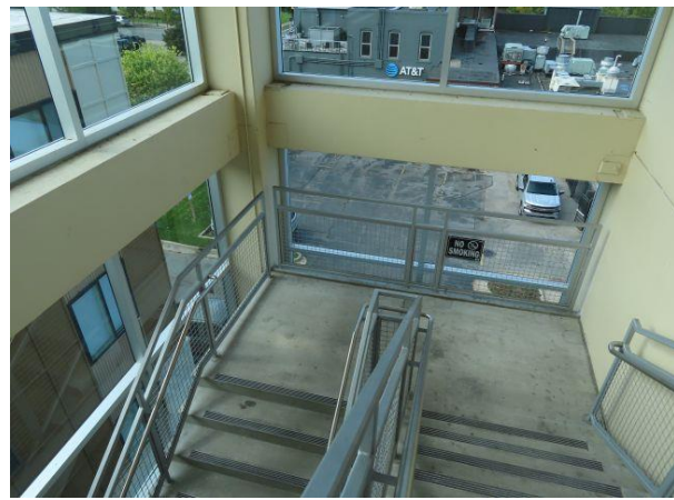
Stair Tower — Stair tower landing southwest stair tower.
