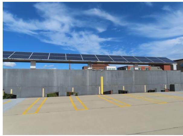
Solar Panels on North End of Structure — North spandrel wall on Level 4 has solar panels mounted at the top of the wall.
