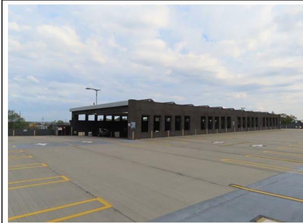
Solar Panels on East Bay Roof — Another photo of the roof and solar panels at the east bay of Level 4.
