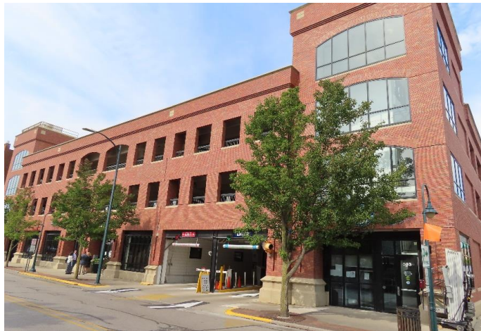
Larry C Hardy Parking Structure
