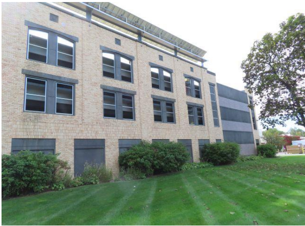
North Facade — North façade of the structure. On the Roof Level you can see one of the solar panels.
