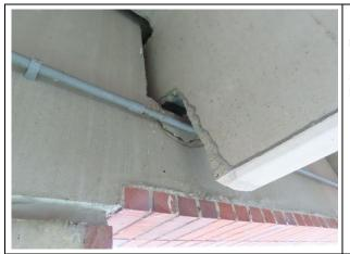
Loose Concrete and Concrete Beam Deterioration — Loose concrete was observed at this location. We recommend all loose concrete be removed and concrete beam deterioration repaired.
