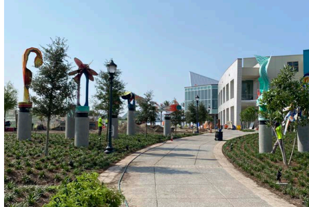
Planted pathway area under construction, expected to be complete in 2024.
